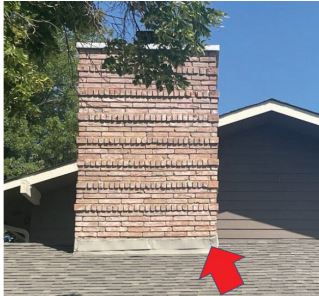
Figure 33. Example of observed gaps at chimney-to-roof joint.
