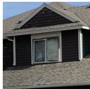
Figure 5. Example of glazing system failures.
