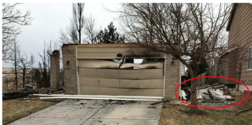
Figure 55. Sample evidence of combustible fencing attached directly to single-family residences in Louisville, Colorado, and serving as a fire pathway to an adjacent home.
