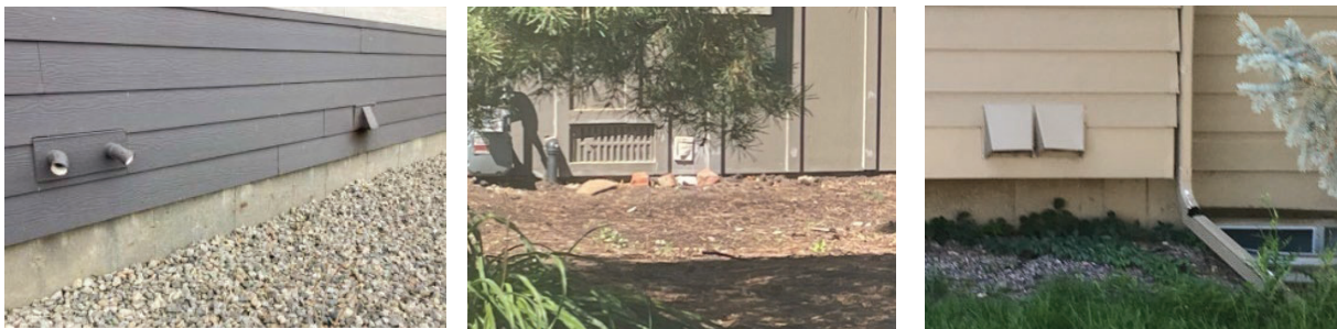
Figure 43. Lack of vent protection in exterior walls, crawlspaces, and basements in Superior and Louisville, Colorado.
