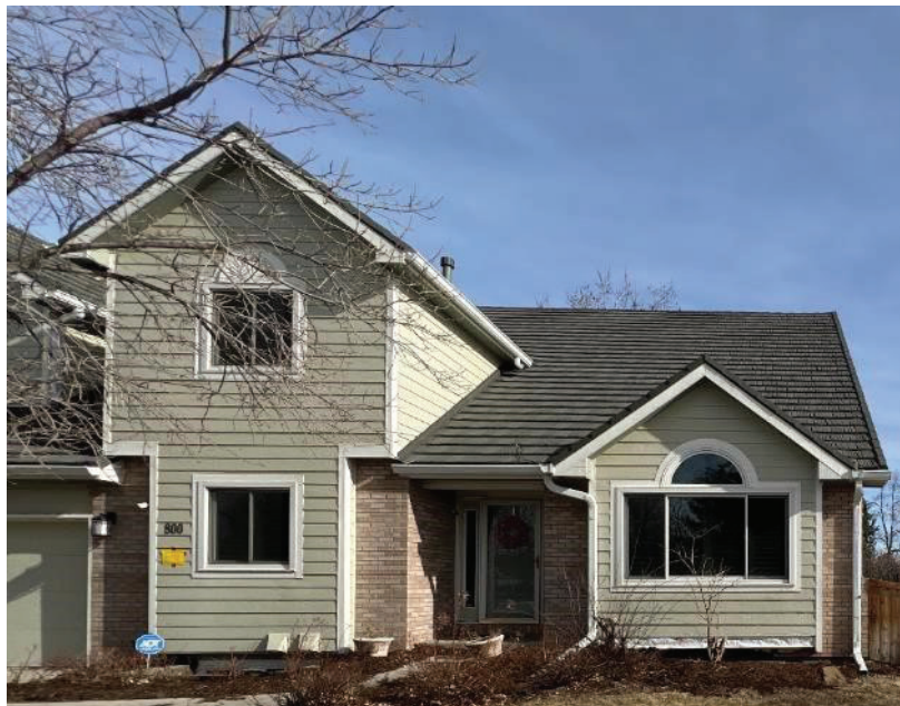
Figure 26. Typical roof system in the Boulder, Colorado area. Roofs tend to have multiple levels, peaks, gables, and joints where debris can accumulate and be ignited by embers.
