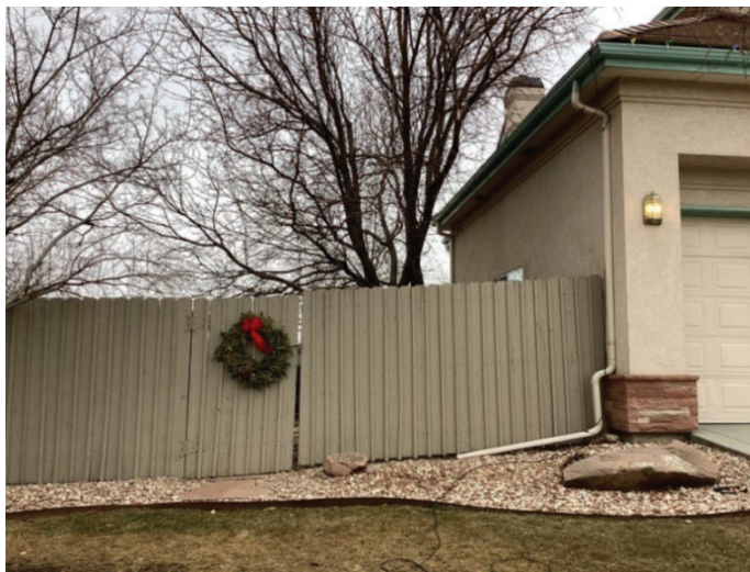
Figure 52. Combustible fencing directly attached to a single-family residence in Rock Creek Ranch in Superior, Colorado.
