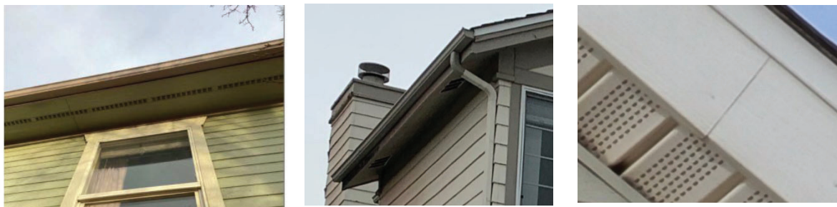
Figure 37. Observed vent protection for soffit eave vents in Superior and Louisville, Colorado.
