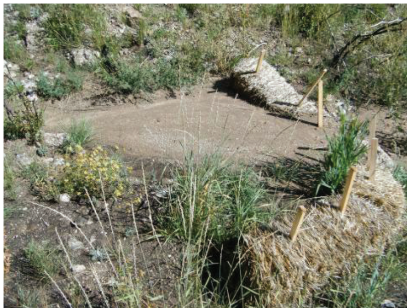
Figure 17. Straw bale check dams can reduce post-fire runoff from steep channels by capturing sediment during rainfalls (USDA Forest Service photo by Pete Robichaud, n.d.).
