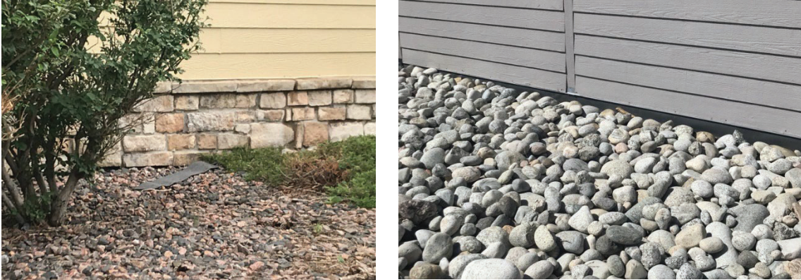
Figure 20. Examples of noncombustible separation at bottom-of-wall-to-foundation joints (Left: noncombustible separation, right: metal flashing).
