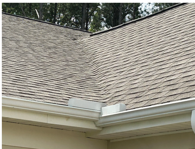
Figure 31. Example of a woven valley.
