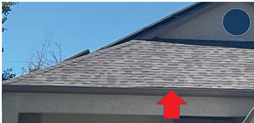
Figure 36. Example of observed vulnerable areas where metal flashing could provide additional protection.
