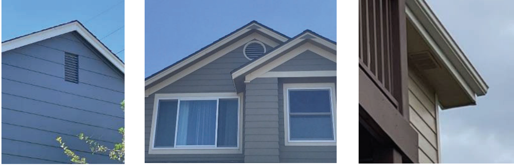
Figure 27. Lack of vent protection in attic vents, gabled roof attics, and soffits in Superior and Louisville, Colorado.
